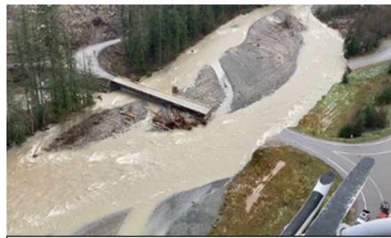
Figure 3 - a bridge washed away at Carolin Mine interchange with Coquihalla Highway 5 near Hope, B.C. due to extreme flooding during November of 2021. (photo from Baum et al. 2021)
